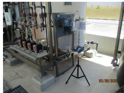
ABPR4_Chemical Dosing (Cooling Tower 40)
